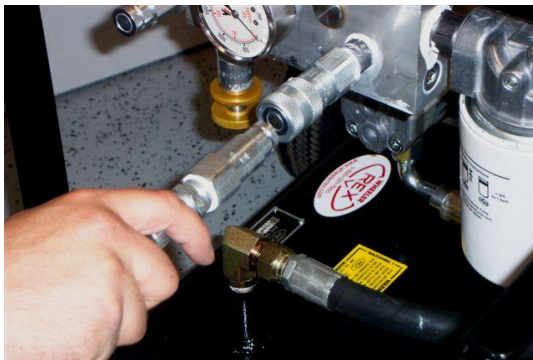
Lines being attached to the Power Pack
